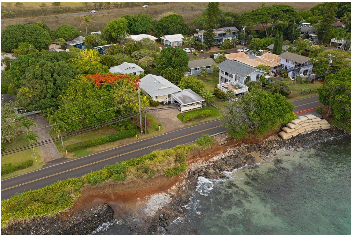
Figure 11: Temporary Repair of a Section of Lower Road at Ka'opala, July 2020
